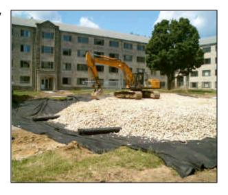
approximately 40% void space in the beds. Here the rainwater is temporarily stored while it infiltrates back into the undisturbed soil below the beds. In extreme events when the capacity of the storage beds is exceeded, flows are permitted to exit the site and flow out the original storm sewer system.
